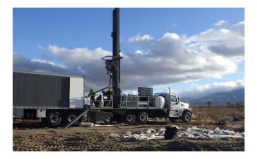
A 400-foot borehole was advanced using rotosonic drilling methods to obtain reliable lithologic information, and a dry monitor well was installed to identify potential water perching during future recharge events. A regional water table monitor well was installed using air rotary casing hammer (ARCH) drilling methods to a depth of 650 feet.
